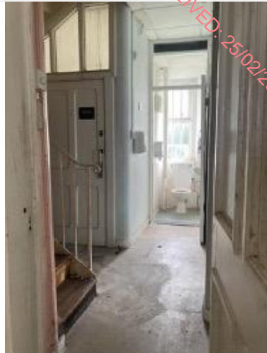
Plate 255: Arrangement of original paneled doors and transom lights within secondary stair enclosure.
