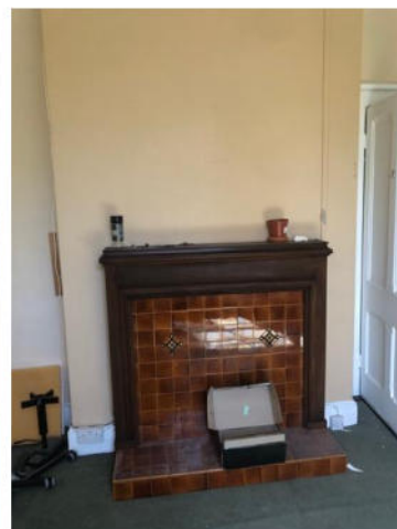
Plate 193: Stepped cornice and picture rail in ground floor accommodation. Timber chimney piece with glazed tile insert.
