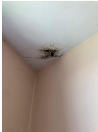
Plate 161: A typical dormitory. Exposed services.
