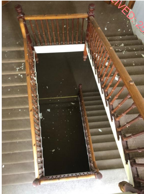
Plate 283: View down central stair
