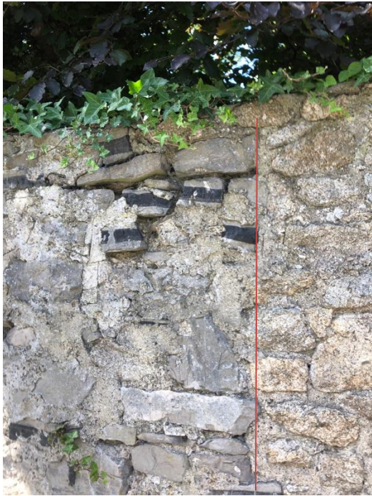
Plate 75: Example of reconstruction of previously collapsed section of wall by others
