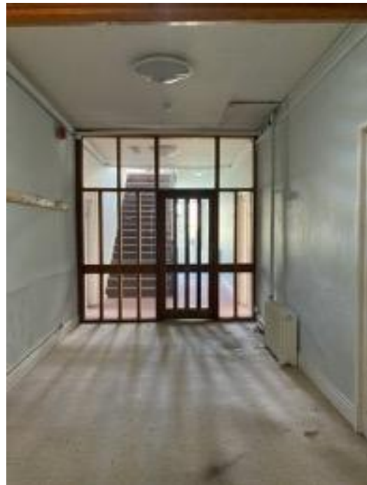
Plate 237: Lower ground floor, fire-rated screen in front of timber stairs in north-eastern bay.
