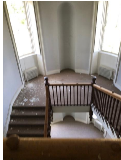
Plate 287: Level 2 landing facing north.
