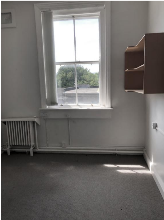
Plate 178: Rear southwestern room at second floor level
