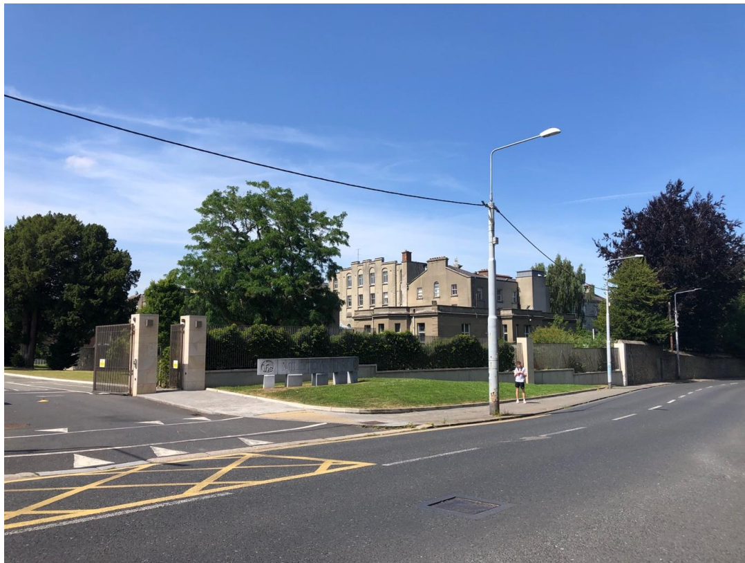
Plate 80: View of range of buildings on site looking north west down Milltown Road
