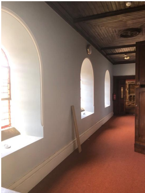
Plate 309: Detail of timber panelled ceiling.
