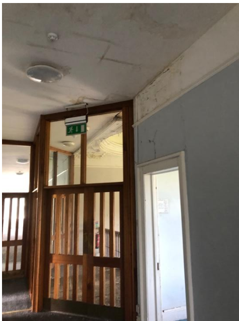
Plate 264: Second floor corridor with later screen doors to central stair and across corridor. Bedroom doors are panelled with moulded architraves.
