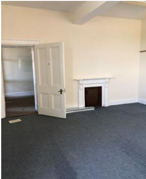
Plate 139: Lecture room within rear extension block at 1 st floor level
