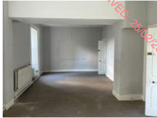
Plate 223: Amalgamated room facing, opposing view.
