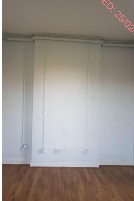
Plate 215: Chimneypiece removed. Contemporary services surface mounted throughout.
