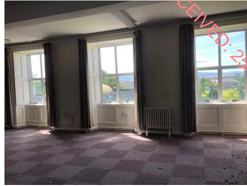
Plate 165: Same Lecture room, view towards two-over-two sash windows.
