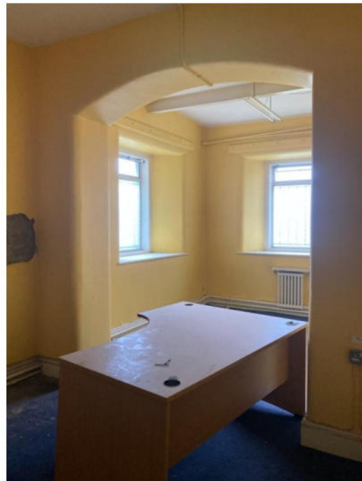
Plate 301: Arched openings supporting columns in Chapel above. Contemporary windows.
