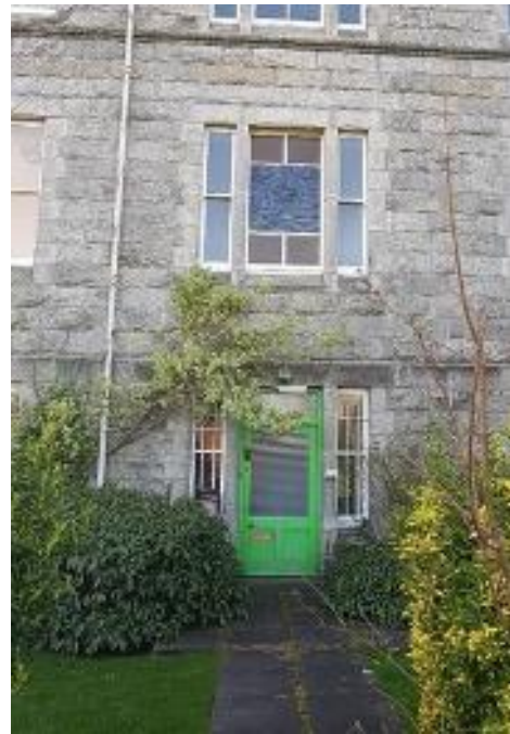
Plate 30: Side door of Tabor House with stained glass on first floor, a later modification
