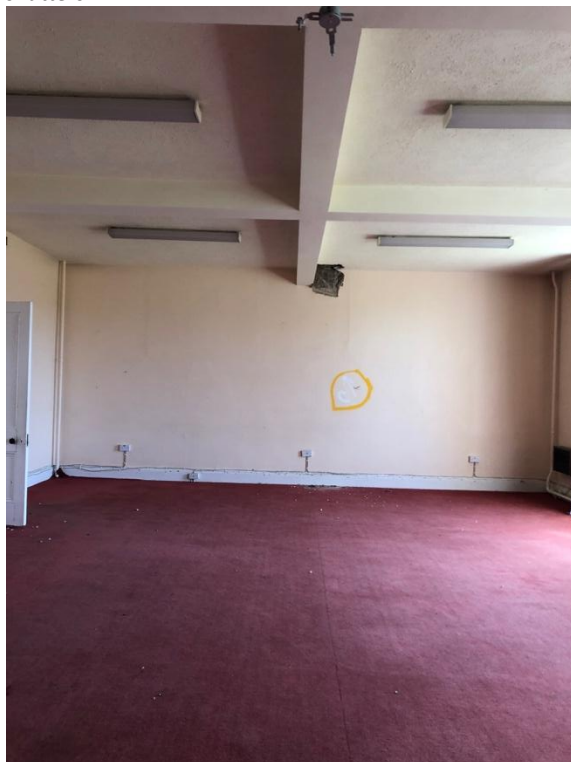
Plate 144: Exposed structural grid in rear extension.
