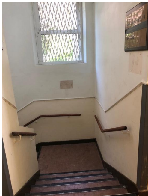
Plate 315: Contemporary stairs to basement
