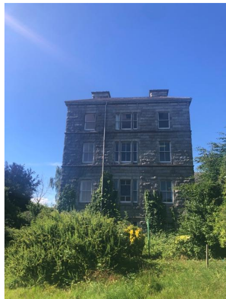
Plate 26: North-east gable of Tabor House in context
