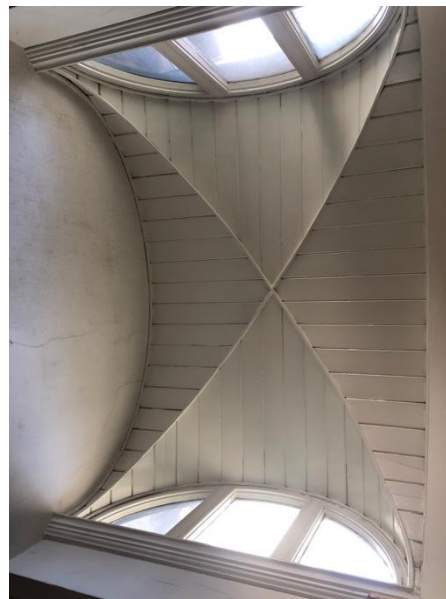
Plate 321: Clerestory light above boarded groin vault
