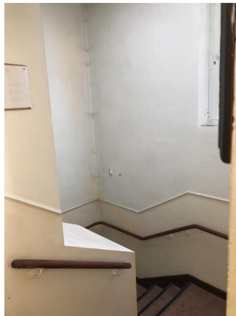
Plate 316: Contemporary stairs to basement.
