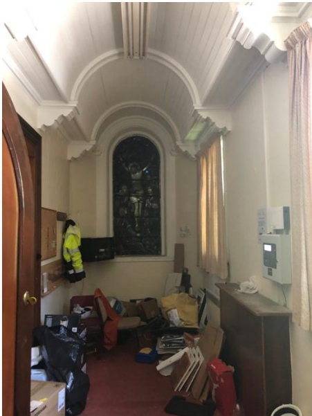
Plate 87: Vestibule/Holy Rosary Chapel, due north towards the apse and stained glass window
