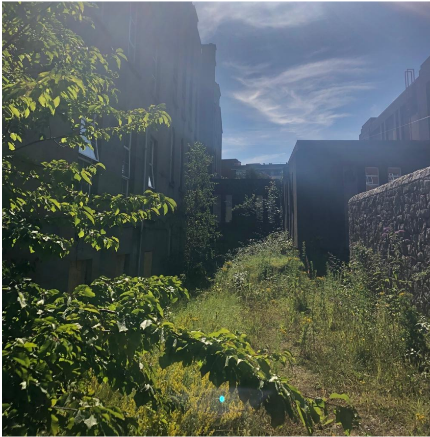
Plate 62: NW elevation of Archive wing where it joins the Rear Extension of Milltown Park House. This is the only point of entry which is internally via Milltown Park House and involves a series of level changes
