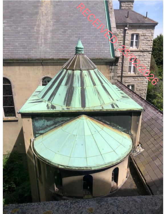
Plate 45: Copper Roof of sacristy, building D2, with slate roof of link building in foreground.
