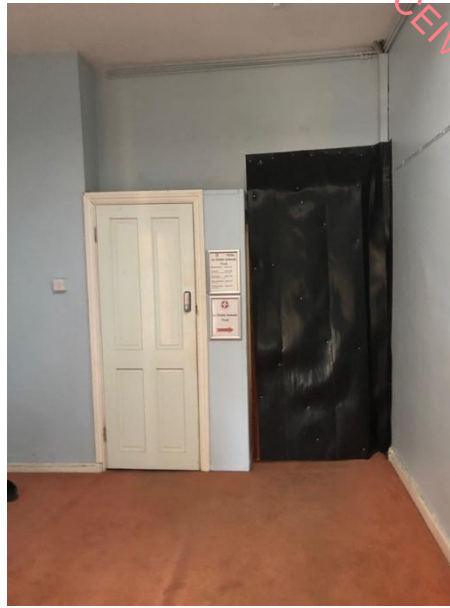
Plate 119: Central hall at 2 nd floor level linking to rear extension block. Note water tank room to lhs of image which extends up into roof void
