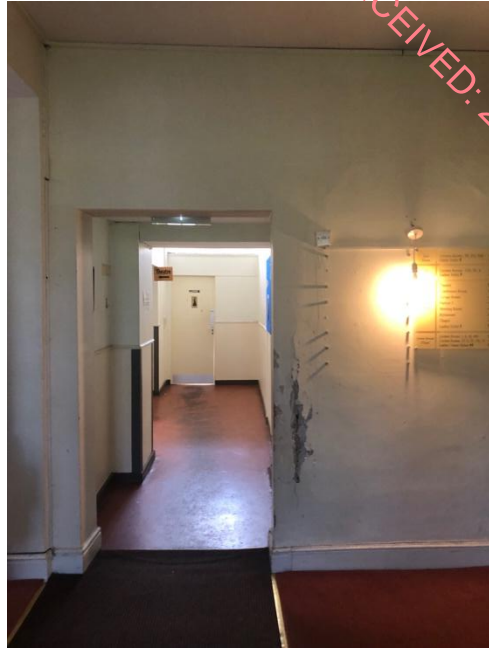
Plate 94: Link within same extension connecting the reception area to the Finlay Wing
