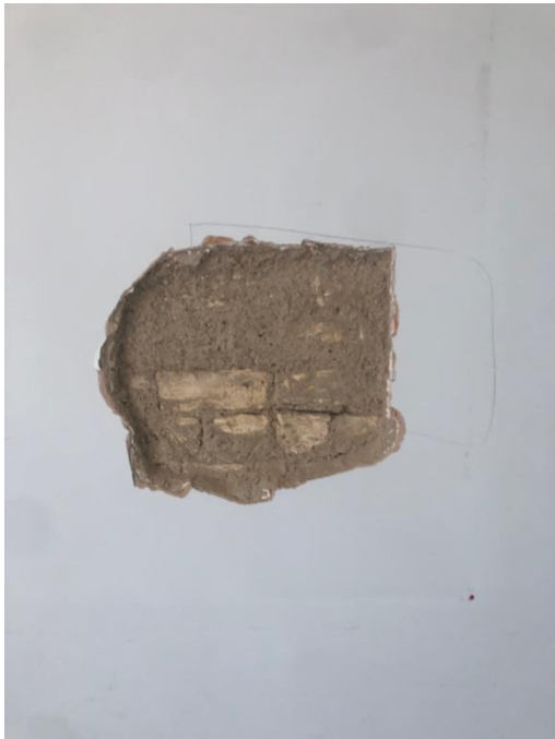
Plate 196: Section of plaster removed to reveal brick substrate.
