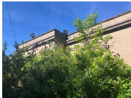
Plate 49: View of Finlay wing, south west from the main entrance
