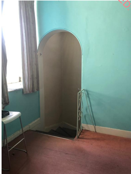
Plate 101: Archway leading to stairs to entrance level
