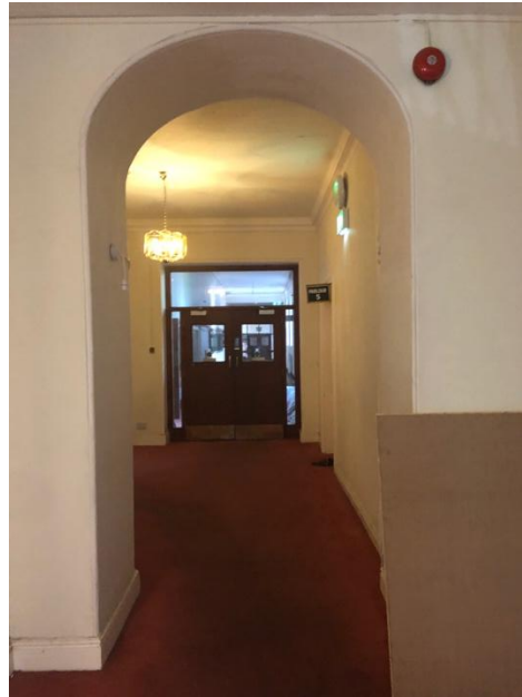
Plate 92: Connection with rear extension block, from rear of entrance hall, with dormitories and study rooms on either side of hall
