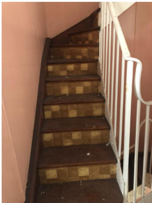
Plate 256: Detail of metal balustrade.
