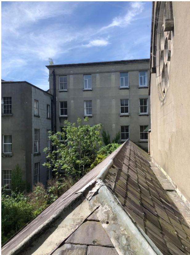
Plate 7: Upper floors of rear (west) elevation of Building A in background, with roof of link building to Chapel in foreground.
