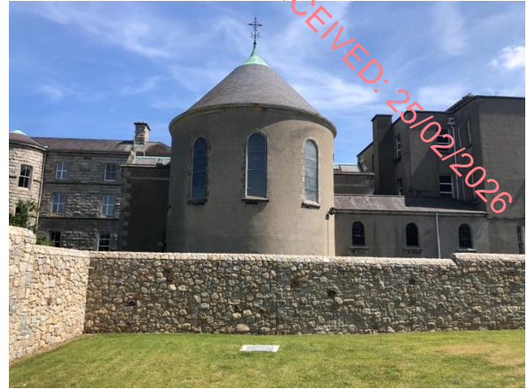
Plate 37: Rear of Chapel, copper turret, with rock-faced granite lower floor and adjoining link building, with dressed window surrounds, image taken from within Gonzaga College grounds with recently erected wall in foreground.
