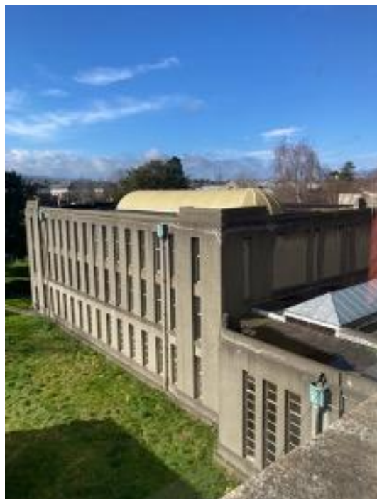
Plate 64: View of SE elevation of archive, as viewed from the rear extension to MPH
