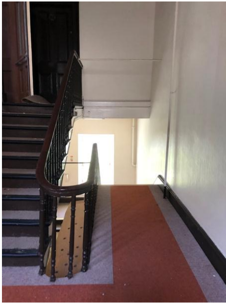
Plate 149: Stairs to rear of former chapel accessing the chapel ante-room
