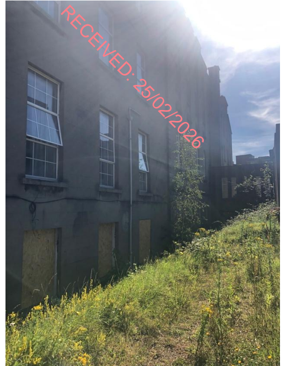
Plate 15: The rendered south elevation of the rear extension
