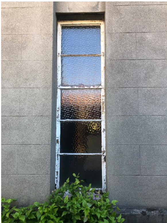
Plate 67: Detail of metal framed casement windows
