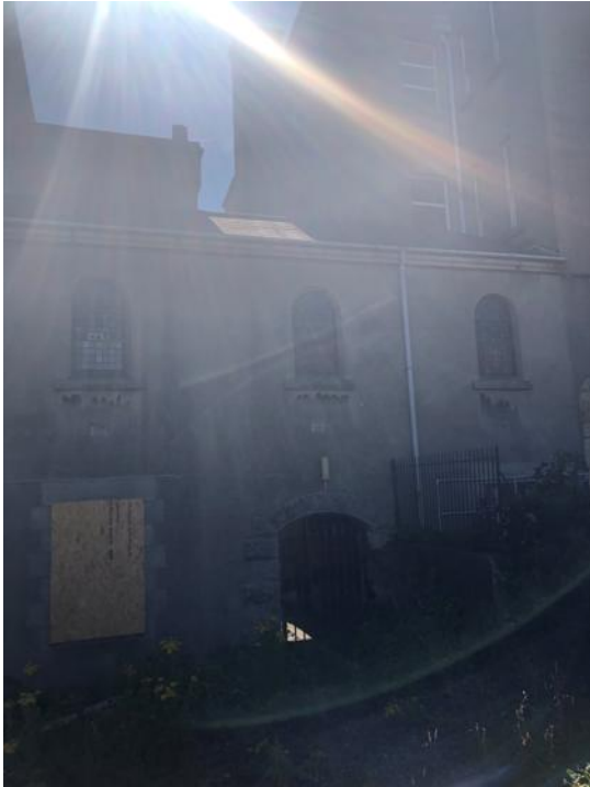
Plate 40: Gated opening to central courtyard at rear of lining structure, between Chapel and rear extension
