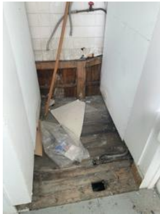
Plate 277: Simple white wall tile laid in stacked bond on wall of former bathroom. Floor tiling removed.
