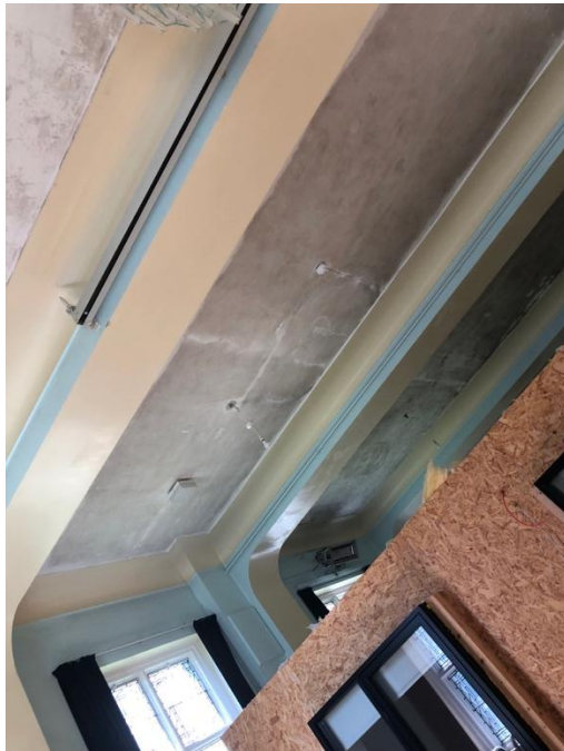
Plate 323: Coffered ceilings formed by structural beams and simple plaster coving.
