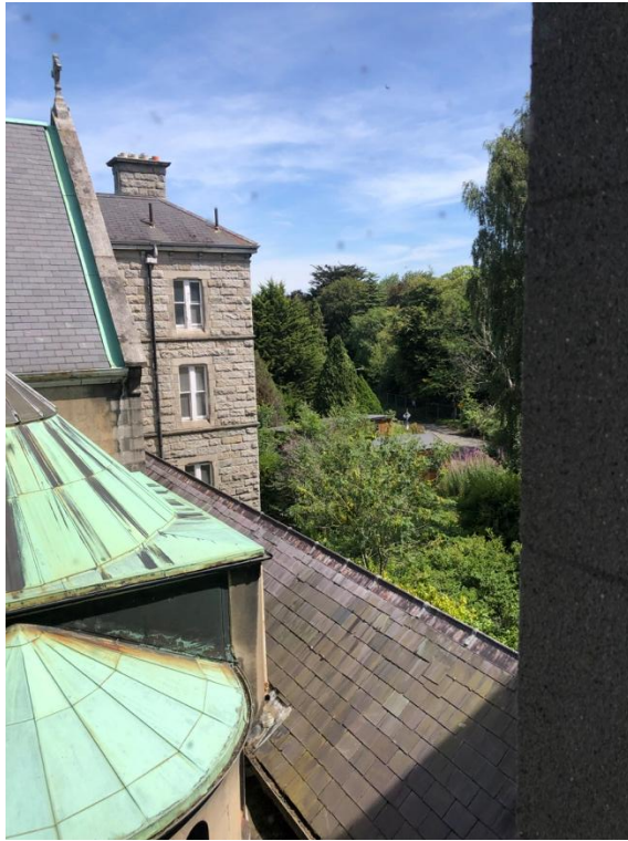
Plate 44: Copper Roof of sacristy, building D2
