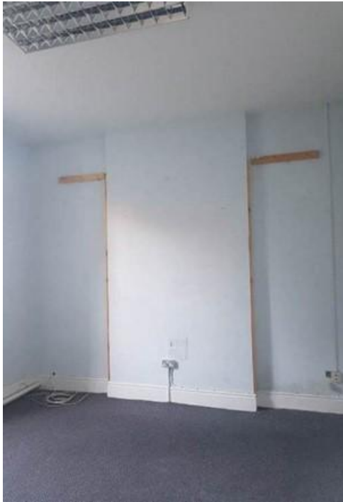
Plate 214: Lecture room, with chimneypiece removed. Contemporary services surface mounted throughout.
