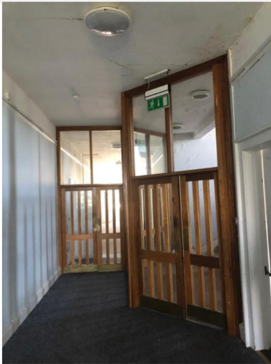
Plate 242: Central corridor with later fire-rated screens across corridors and enclosing stairs.
