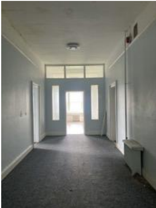
Plate 270: Fire rated partition door with glass panels within central corridor
