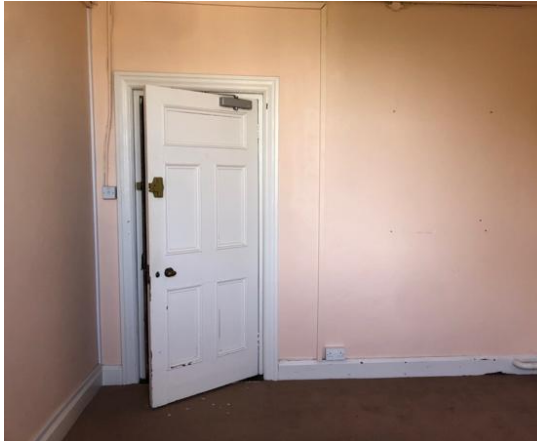
Plate 160: A typical dormitory in main corridor with modern door and architrave. Exposed services.
