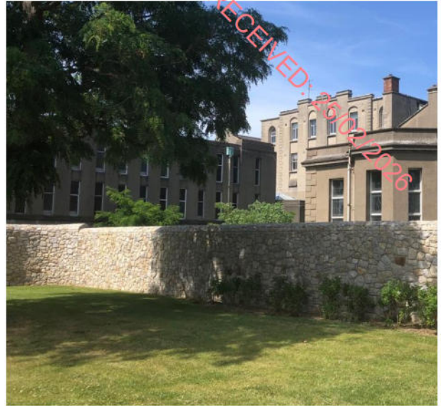
Plate 58: SE elevation, Finlay wing in foreground
