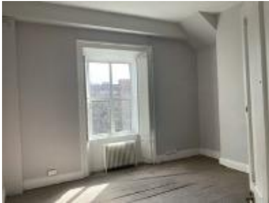
Plate 274: Original window joinery.
