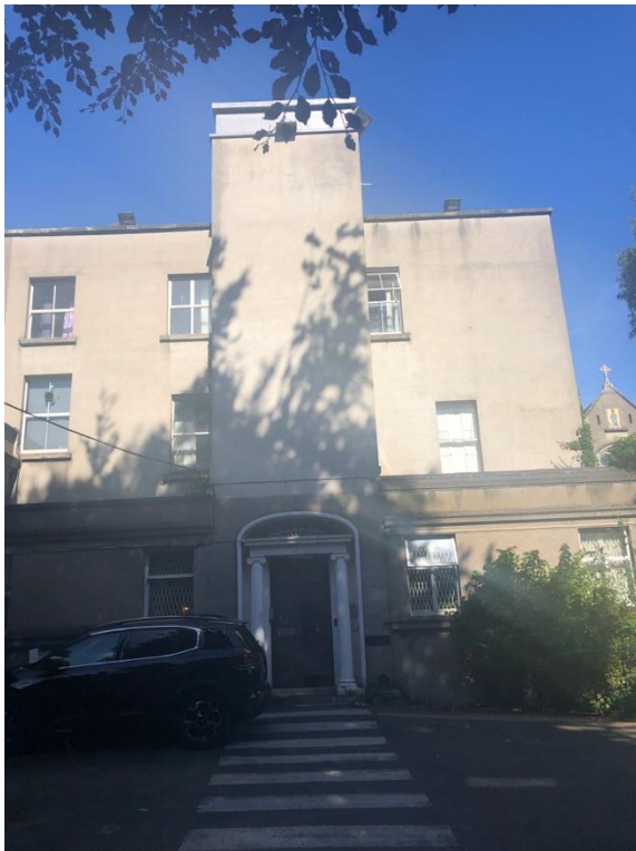
Plate 1: Milltown Park House entrance with some of its many extensions visible
