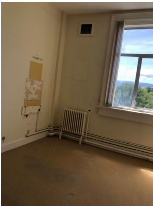
Plate 162: Larger dormitory room with modern windows, contemporary wall linings.
