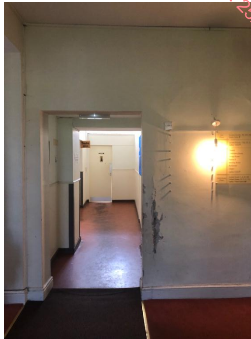
Plate 314: Escape route from same entrance
