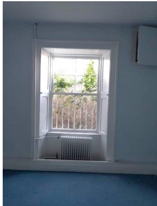
Plate 217: Lower ground floor two-over-two timber sash window with panelled shutters.
