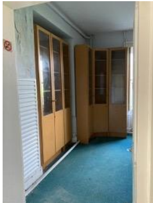
Plate 241: Contemporary fixtures and fittings and services. Exposed services.
