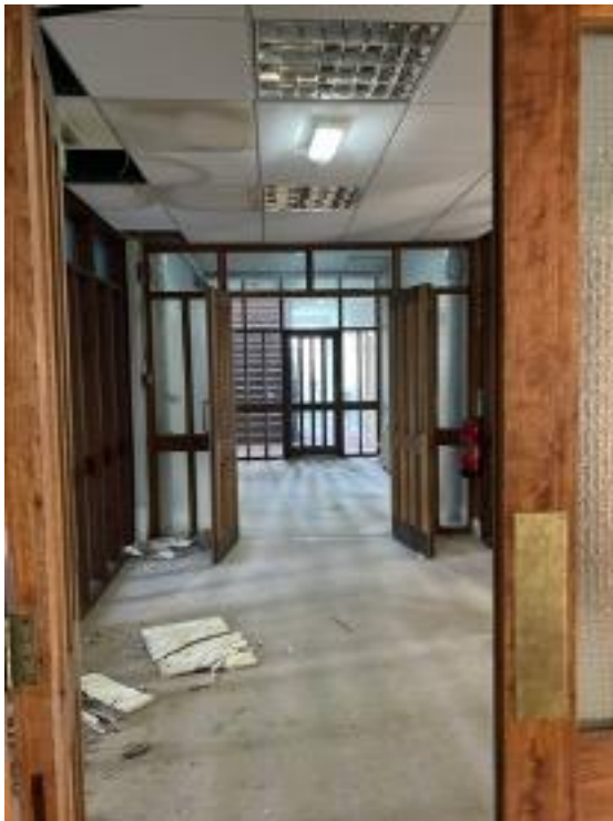
Plate 236: Later lobbies and cross-corridor fire rated screens and suspended ceilings.
