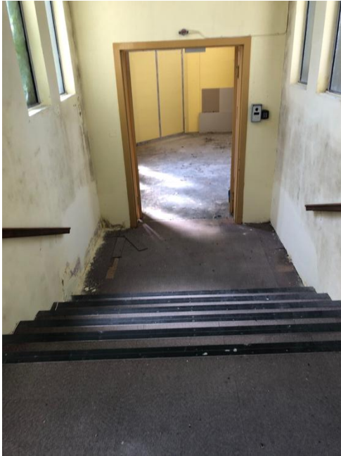
Plate 367: View towards entrance to archive. Note multiple level changes.
