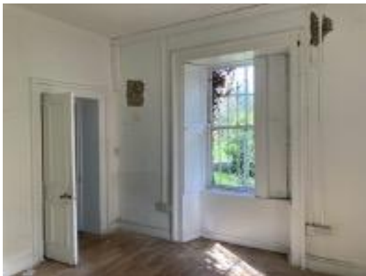
Plate 212: Original door and window joinery. Localised removal of internal render to inspect underlying masonry fabric.
