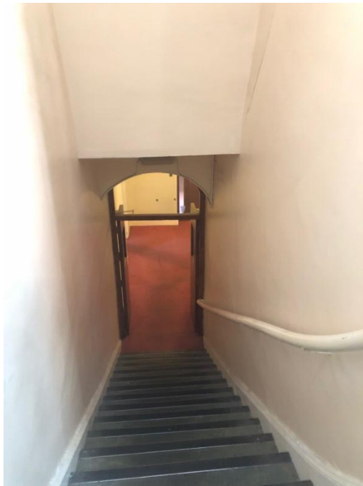
Plate 85: Later stair to 1 st floor from rear of reception area
