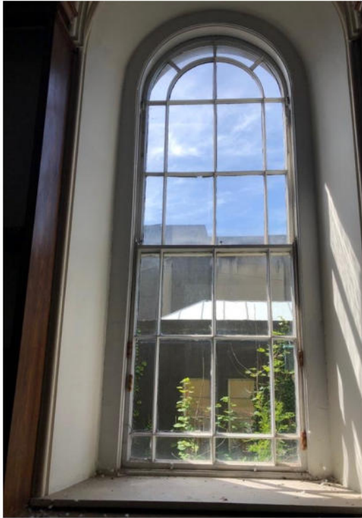
Plate 153: Round headed timber sash window with margin lights within former domestic Chapel.
