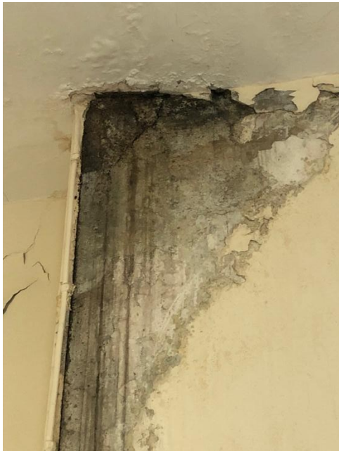
Plate 120: Opening up investigations to uncover brick substrate.
