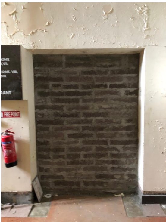
Plate 132: Blocked up former link to Community Building, outside the subject development site
