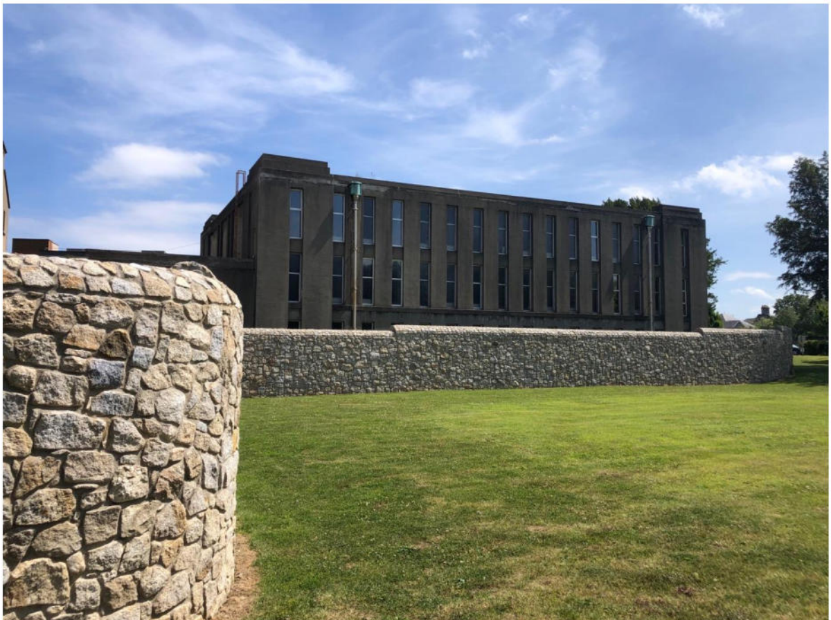
Plate 59: SW elevation of archive
