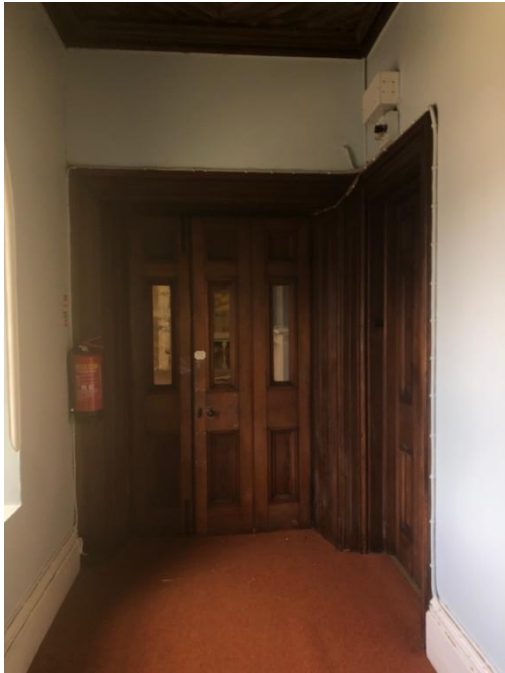
Plate 311: Doorcase from Chapel (left) to sacristy (right) within Building B2
