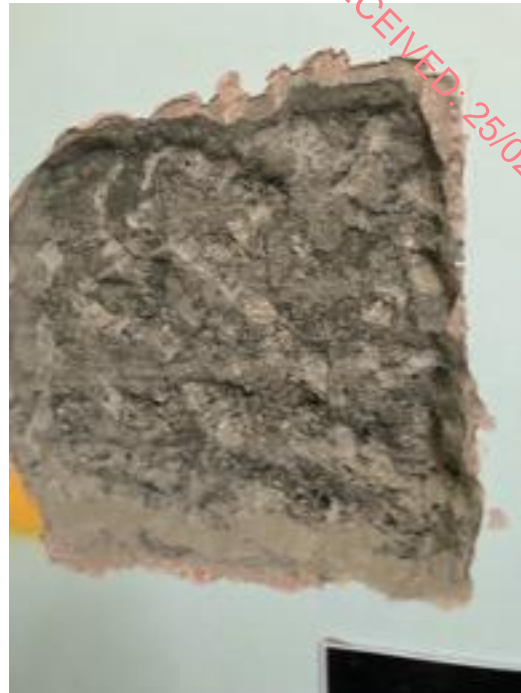
Plate 322: Localised area of render removed to reveal masonry substrate.
