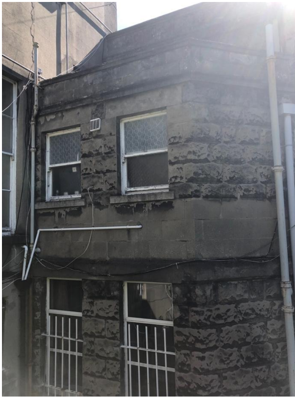
Plate 53: View of NW elevation of Finlay wing and awkward connection to Milltown House. Note stained window panes dating from post 1949 reconstruction
