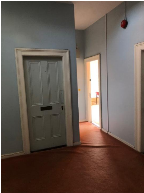
Plate 118: Internal circulation within the uppermost level of Milltown Park House
