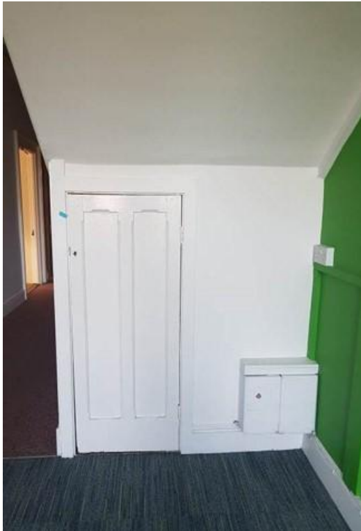
Plate 210:: Under stair cupboard in hall at side entrance. Panel detail matching the entrance door.
