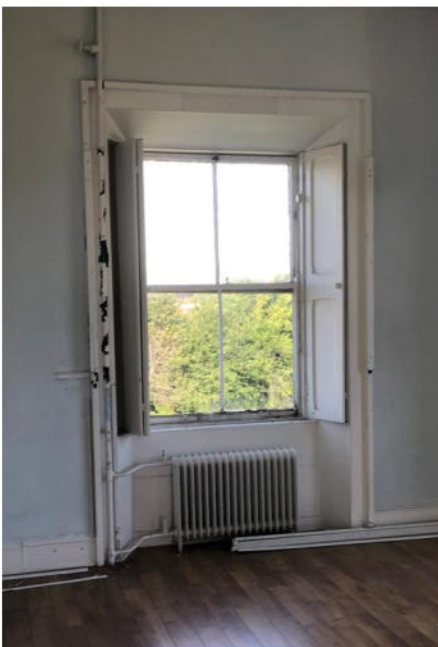
Plate 260: Detail of tripartite sash window.
