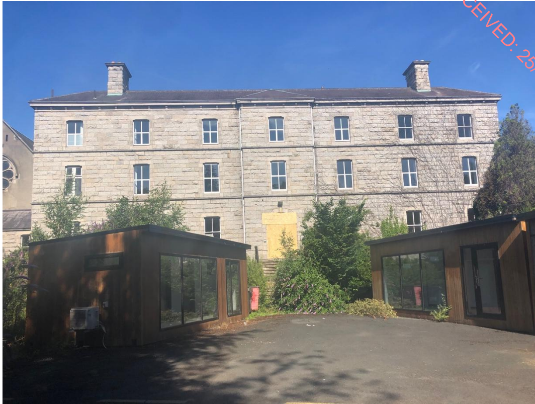
Plate 22: Symmetrical front elevation of Tabor House, a three storey over lower ground floor, 7 bay building. Temporary prefabricated structures in foreground.
