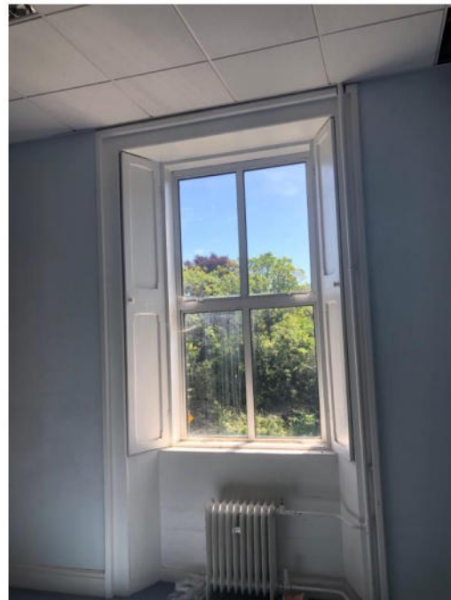
Plate 245: Typical first floor accommodation, original window-box with contemporary uPVC window. Exposed services, no decorative plasterwork.
