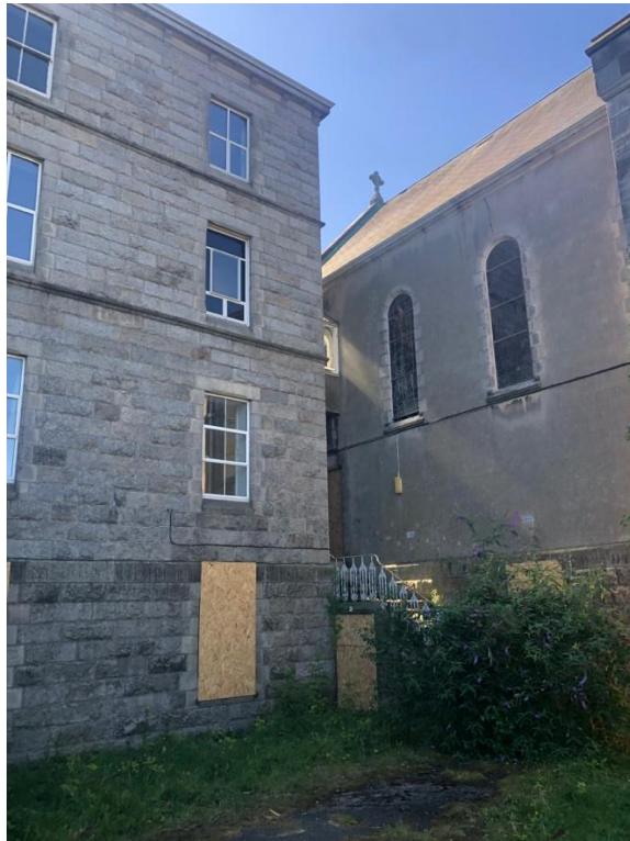
Plate 31: Connection of Tabor House to the later Chapel: comprising a set of stone steps to first floor level, and a glazed link at second floor to the mezzanine at the rear of the Chapel
