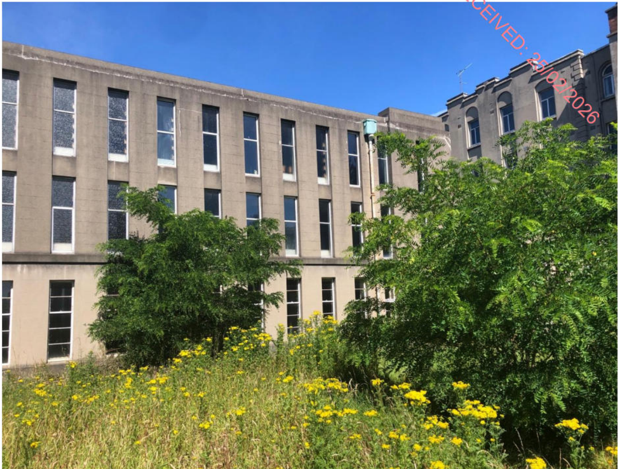
Plate 60: SE elevation of Archive wing. Original 1930's window frames. Copper hoppers to rainwater goods, Art deco detailing of parapet walls
