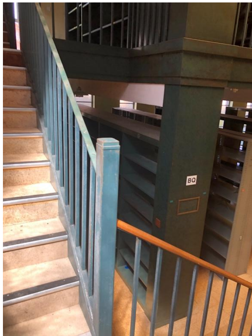
Plate 357: Detail of stair steel banister and oak handrail
