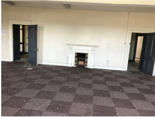
Plate 164: Large lecture room with fireplace at first floor level. Chimneypiece with tiled cheeks.
