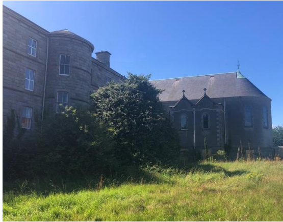
Plate 36: Rear of Chapel with Tabor House in foreground.
