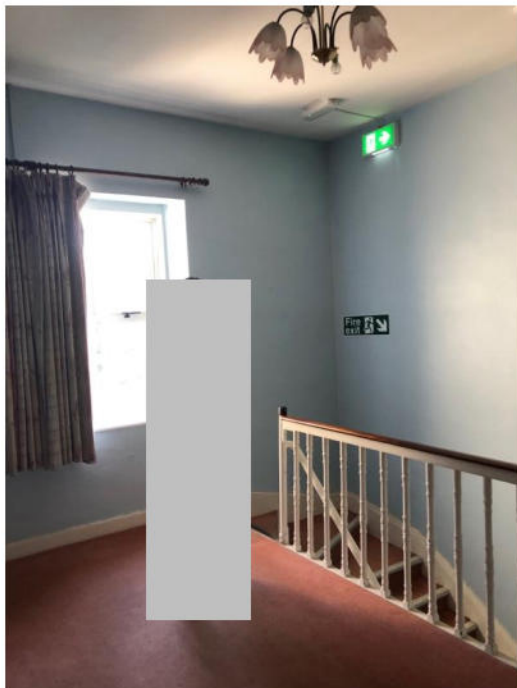
Plate 116: Level 2 landing facing south-east towards front elevation.
