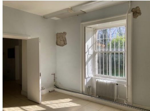
Plate 225: Localised removal of plasterwork to reveal underlying masonry fabric.
