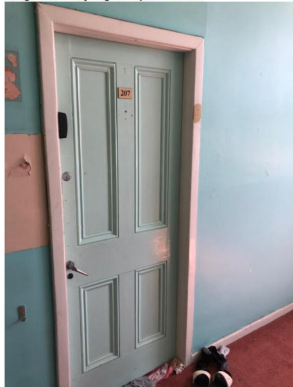
Plate 110: Panelled door to bathroom, projected above main entrance on front, south-east facing elevation.
