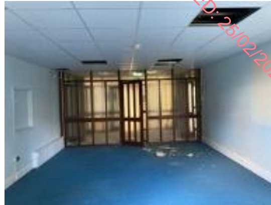
Plate 235: Later timber-framed fire screens within corridor.
