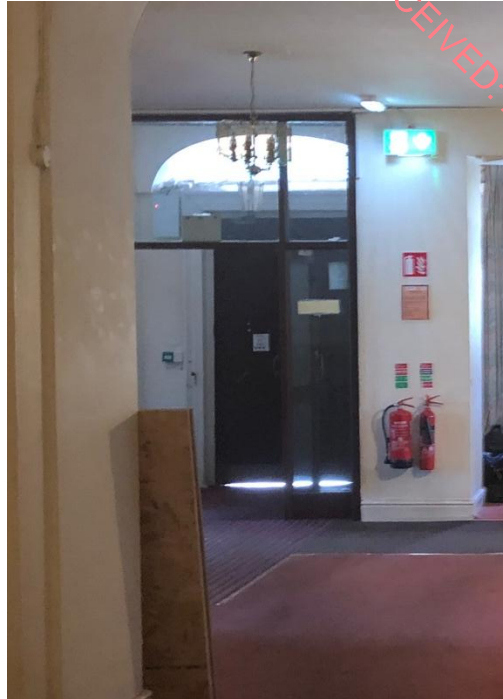
Plate 82: Entrance door of Milltown Park House with cobweb fanlight visible
