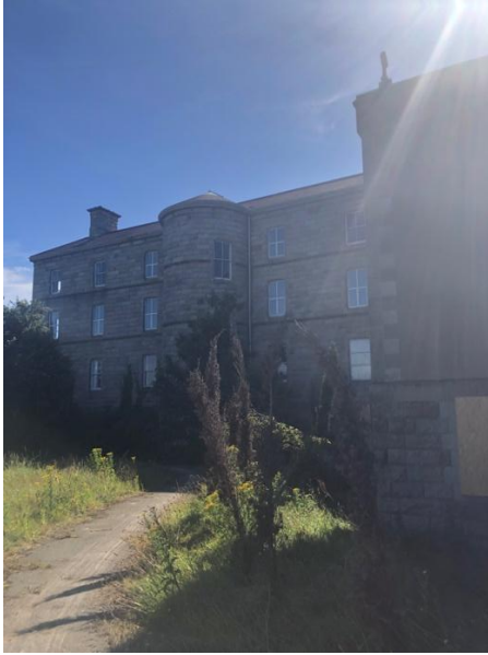
Plate 27: West elevation with bowed bay
