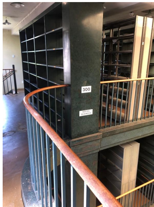
Plate 358: Detail of curved handrail at end floor mezzanine level
