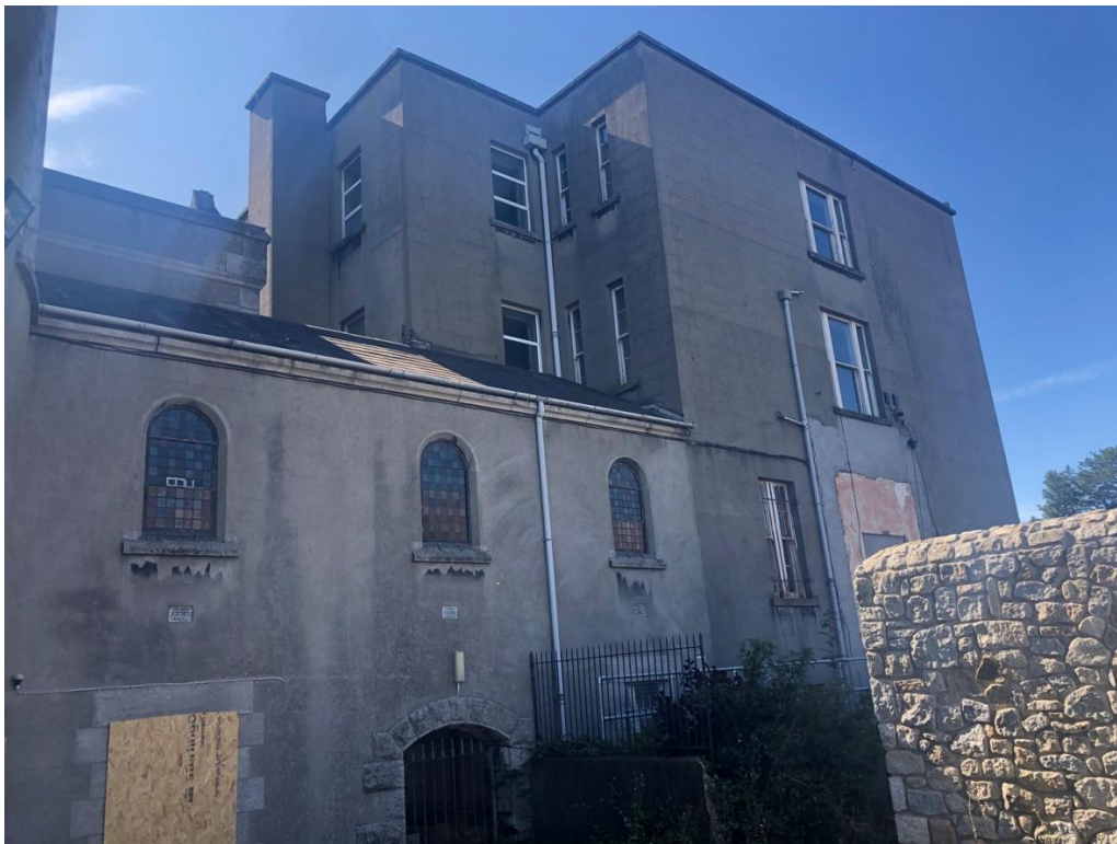
Plate 21: North-west elevation of link between rear of MPH extension and Chapel. Rusticated stone surround to gated passage to central courtyard. New boundary wall, part of recent separation works, in foreground.
