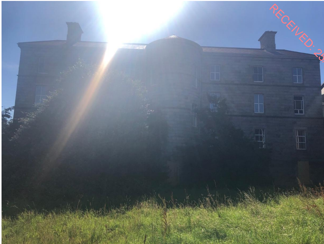
Plate 24: Tabor House rear/west elevation, with bowed bay of central staircase, note the array of fenestration types; the original 2 over 2 sashes being the most prevalent
