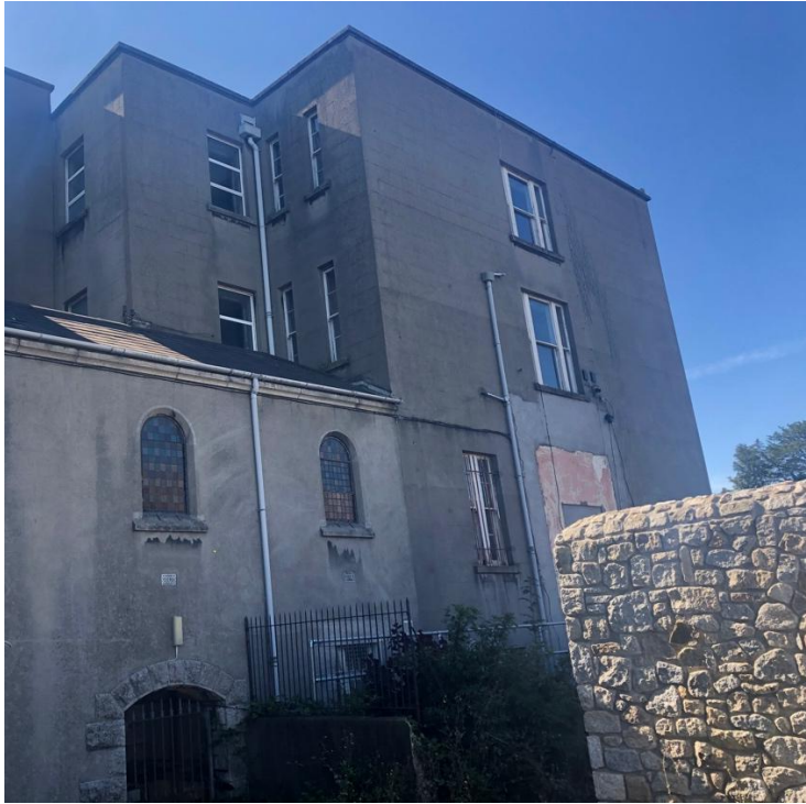
Plate 14: Rear extension with repaired gable following removal of former link structure, recently demolished.
