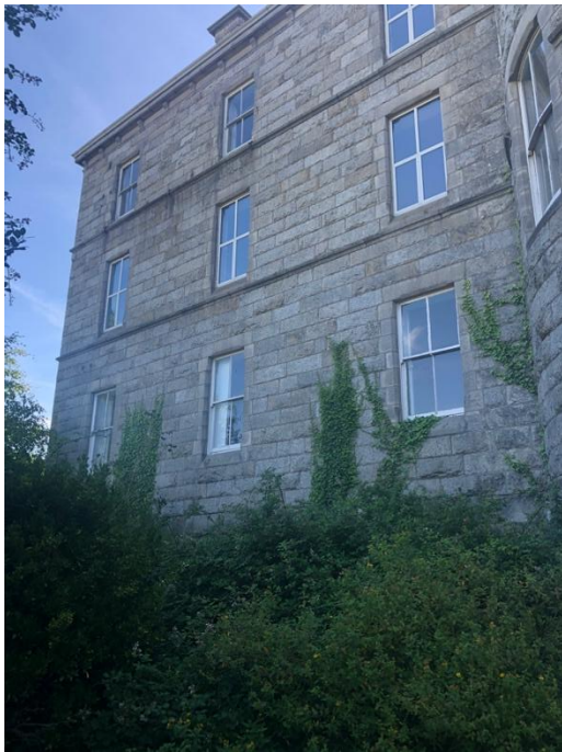
Plate 29: North east gable elevation of Tabor House
